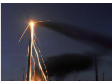
Damage to wind turbine blade
